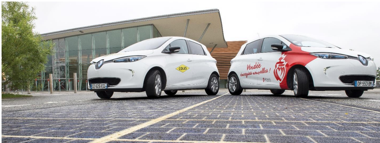
Fig. 8. Wattway's solar modules integrated to serve as a roadway surface [21].
