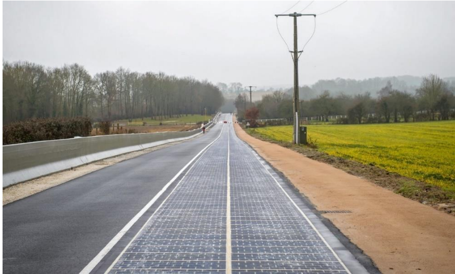
Fig. 6. The world's first photovoltaic road opened in Tourouvre , Orne, France. Route in Tourouvre-au-Perche will be used by about 2,000 motorists a day during two-year test period [28].
