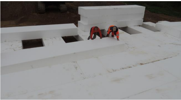
i) Installation of EPS-blocks at sec. 5 (16.9.2015)
