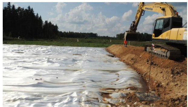
f) Construction of edge barrier at sec. 4. Peat rod in bottom right corner. (12.8.2015)
