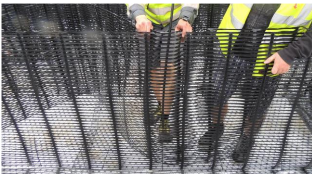
e) Construction of Geocell structure at sec 3. (31.7.2015)
