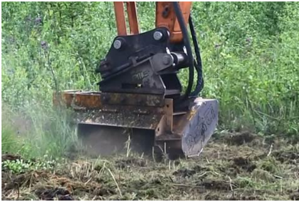
Figure 6. Milling the topsoil (stumps, roots, small sticks, grass etc.) for working platform.
