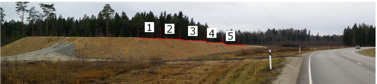
k) Test sections 1-5 after surcharge loading (11.11.2015)
