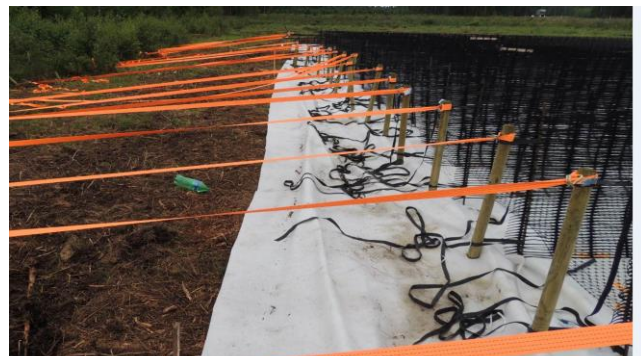
d) Construction of Geocell structure (31.7.2015)
