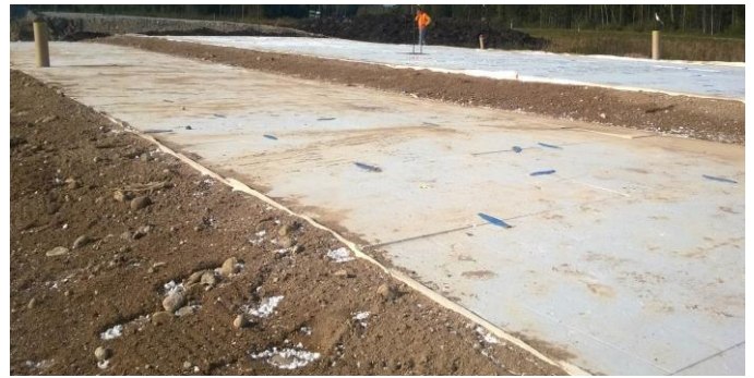
j) Surface of the EPS-layer at sec. 5. Plastic connectors on between EPS-blocks (24.9.2015)
