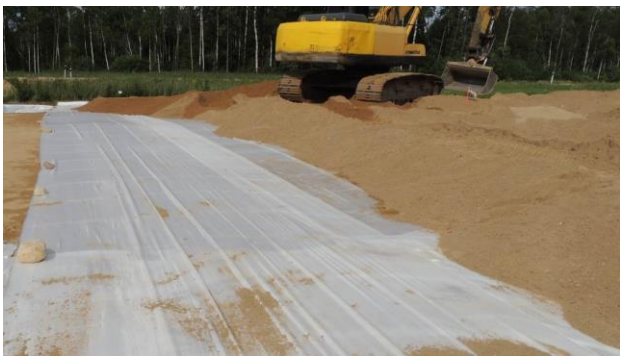
c) Installed upper reinforcement, sec. 2 (21.7.2015)
