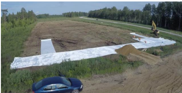
a) Start of construction of sec. 1 (20.7.2015)
