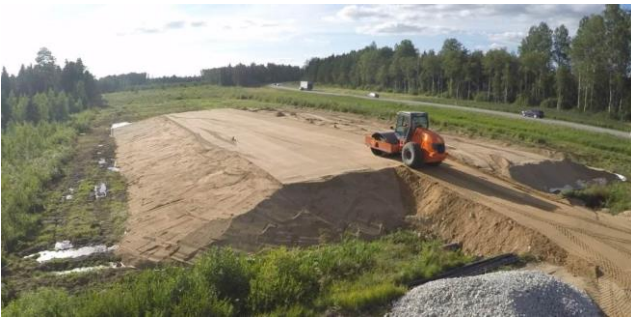
g) Compaction of the embankment. sec.1 (24.8.2015)
