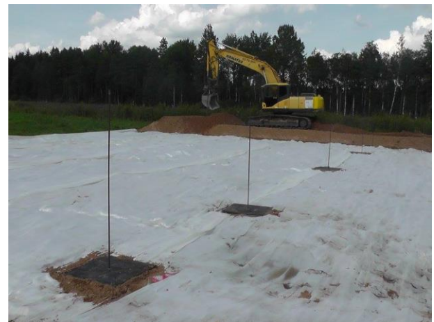
Figure 15. Peat roads placed in pre-designed locations on top of the geotextile-covered peat layer. (Ellmann 2015)
