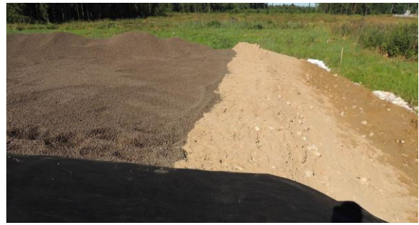
h) Construction of LWA layer at sec 4. (25.8.2015)
