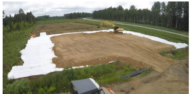
b) Construction of embankment sec. 1 (20.7.2015)
