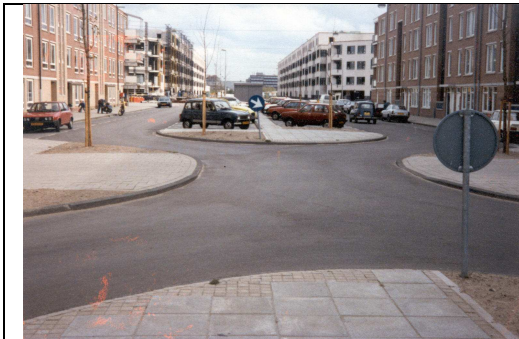
Traffic calming by protrusions
