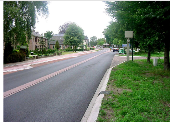
Distributor road: 'median', parking bays, speed camera
