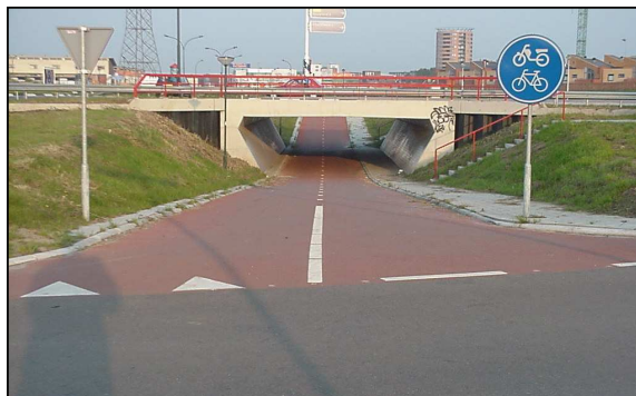
Well-designed split level crossing for cyclists and pedestrians
