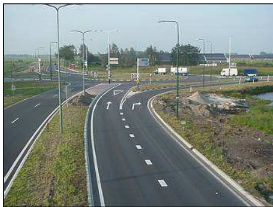
Two-lane roundabout with bypass
