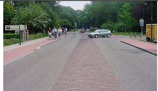
Traffic calming by convex 'median' and narrow lanes
