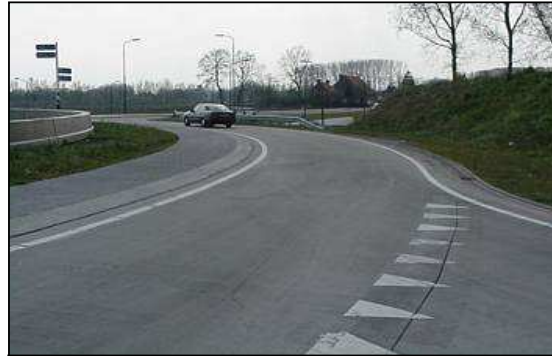
Lane and overrun area of a single lane roundabout
