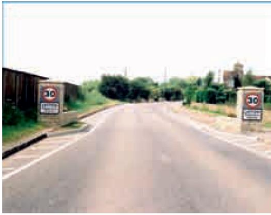
Fig. 3.8 Gateway feature, Latton
